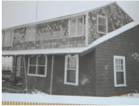
Cottage on Juniper Lane with new addition
